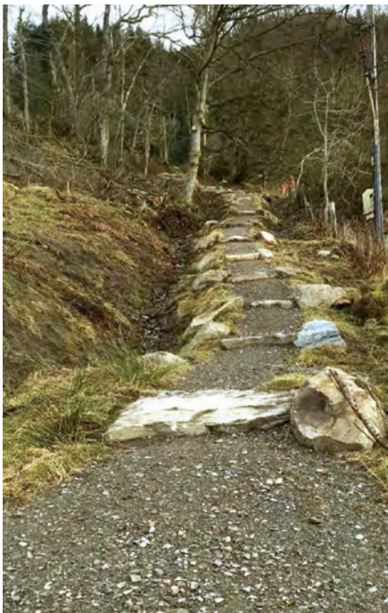
After: Ben A'an Path - Raised path with Anchor bars and water bar features.
