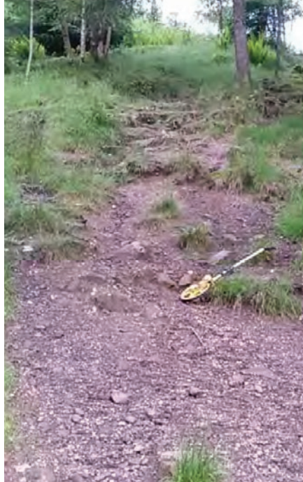
Before: Ben A'an Path - Wide and badly eroded section of path above the bridge. This section is notably steep.
