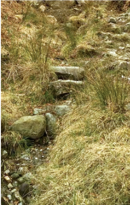
Before: Ben A'an Path - Section typical of collapse and erosion of existing path.
