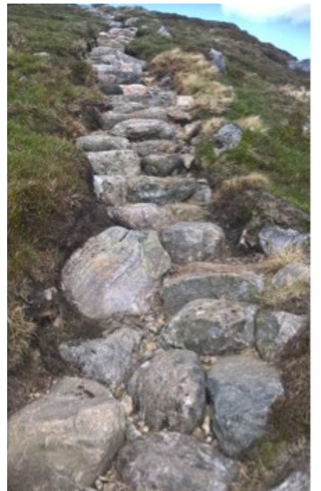
After: The Snub Path Upgrade and Repair.
