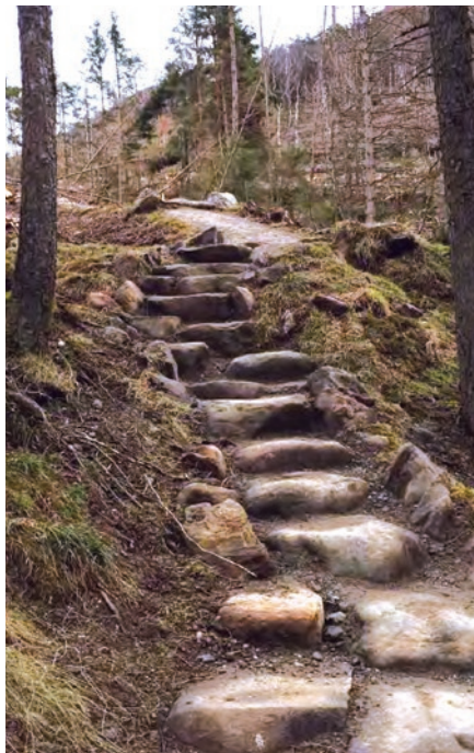
After: Ben A'an Path - Block pitching to address steep incline and outside edge revetment to stabilise embankment.
