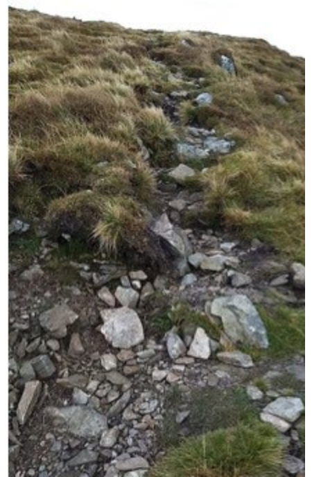
Before: The Snub Path Upgrade and Repair.
