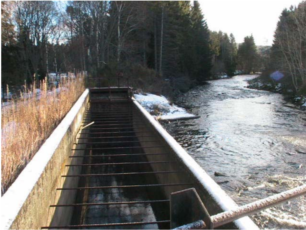
Fig. 3. Existing intake, looking downstream
