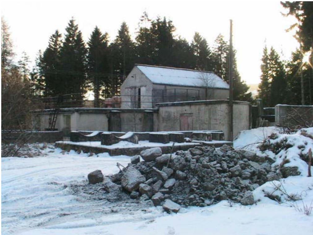
Fig. 4. Existing turbine house – works not part of application
