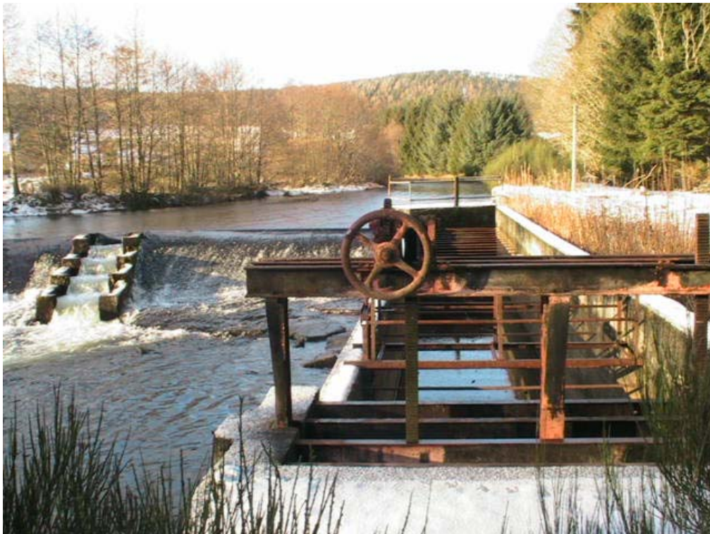
Fig. 2. Existing intake, weir and salmon ladder, looking upstream.
