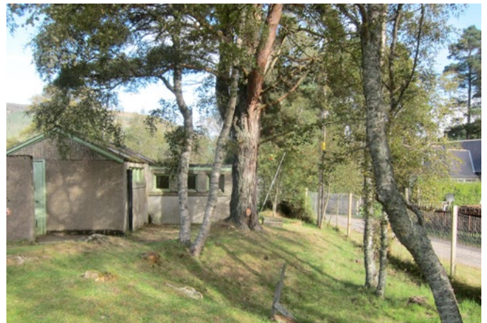
View of Toilet Block with Broombank Terrace at right.
