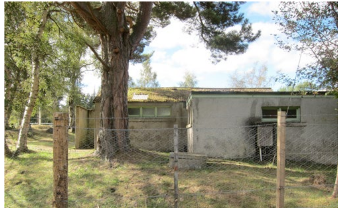
View to the rear of the Toilet Block from Broombank Terrace.
