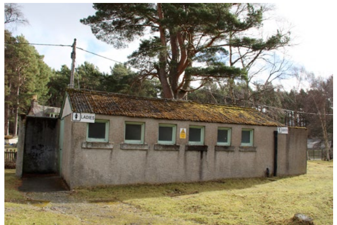
Toilet Block proposed for removal. Scot Pine in background shall be retained.
