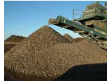
Mobile crushing machine used to recycle demolition waste into aggregate
