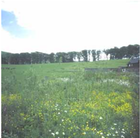
© Living Water Wetland and willow soakaway for the treatment of sewage at a 30-person development at Romanno Bridge near West Linton, Midlothian.
