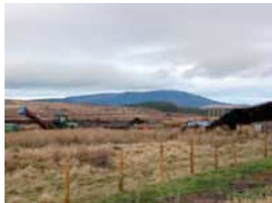
Machinery and stockpiles of excavated peat
