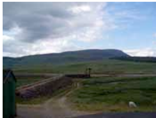
Infrastructure associated with the dam
