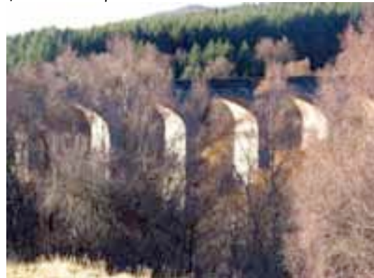
The high arches of the railway bridge over the gorge
