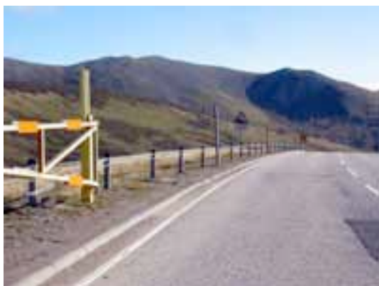
Road side signs, concrete edges and barriers reflecting the high winter use of the road, combine to create visual clutter
