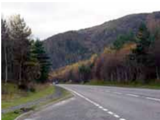
The A9, within cuttings and further enclosed with woodland, and Craigellachie looming into view
