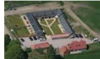
Invertromie Steading Davidson Baxter Partnership Ltd / Ironhorse Developments / Speybuild Ltd Location & completed date Kingussie, April 2016 Category - Commercial
