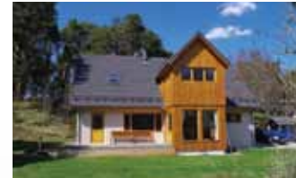
Pine Acre Rona Douglas Interiors Location & completed date Carr-Bridge, November 2015 Category - Residential Extensions & Refurbishments
