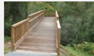
Bridges on Speyside Way Extension Geoff Freedman Rural Bridges (designer) COAT (facilitator) Location & completed date Aviemore to Newtonmore, March 2015 Category - Infrastructure
