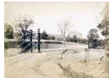
Suspension footbridge at Birkhall
