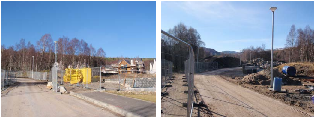
Fig. 2 and 3 : Views towards Phase 4 of the development site
