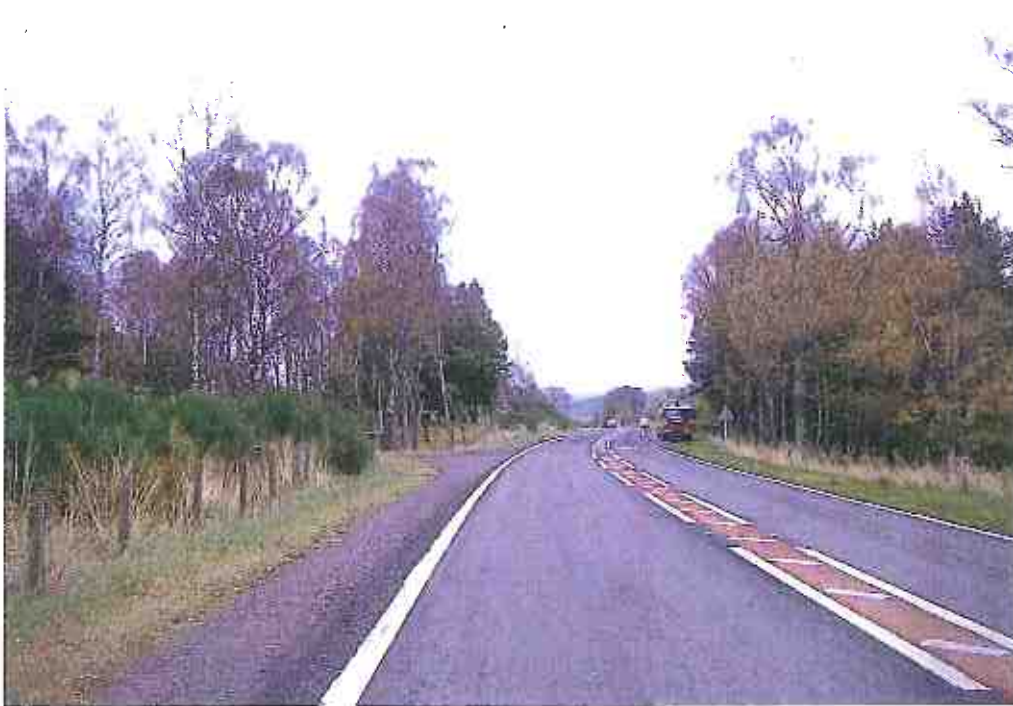
View of existing access from position 215 metres west on eastbound approach
