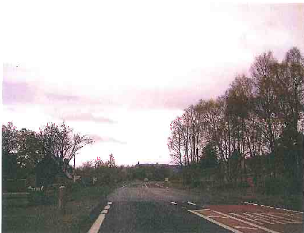
View of existing access from position 185 metres east on westbound approach
