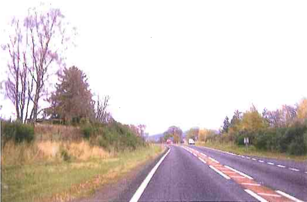
View of existing access from position 100 metres west on eastbound approach
