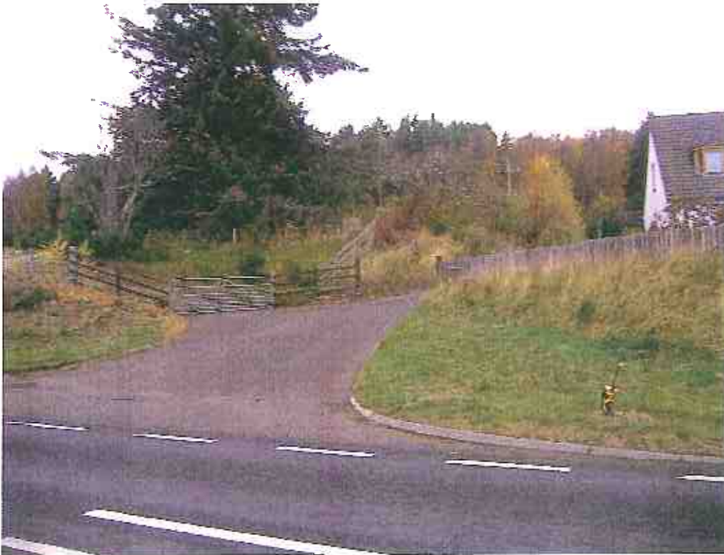
View of existing access from position southeast looking northwest
