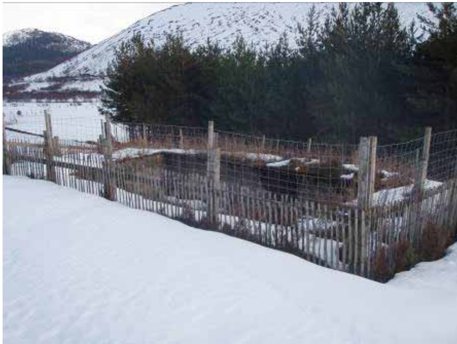
Fig.5 – Photo showing filter bed tank
