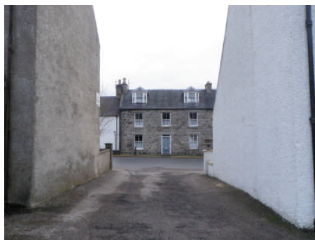
Fig. 9 : Access, as viewed from site
