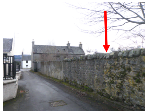
Fig. 4 : Boundary wall to the rear of 2 proposed blocks of flats
