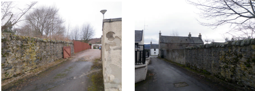
Figs. 11 and 12 – existing boundary treatments on the northern boundary of the proposed site
