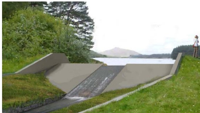
Fig. 12- Reconstructed dam and spillway on Loch Gynack
