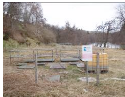
Fig. 5 - Existing WwTW (6 underground septic tanks)
