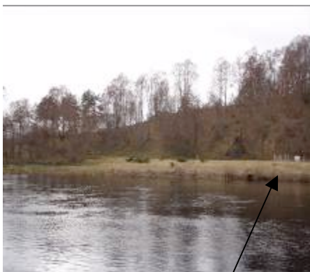
Fig. 4 - Site from opposite bank (Existing WwTW far right)
