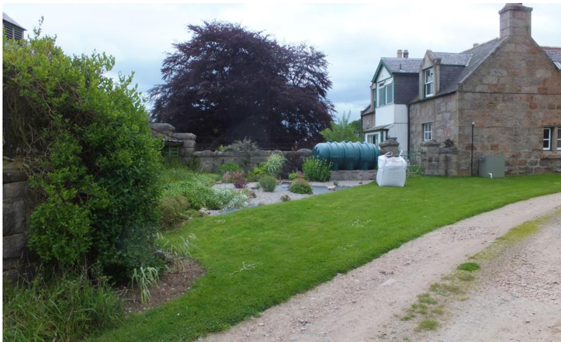
Photo 1 Site Viewed from the Track
