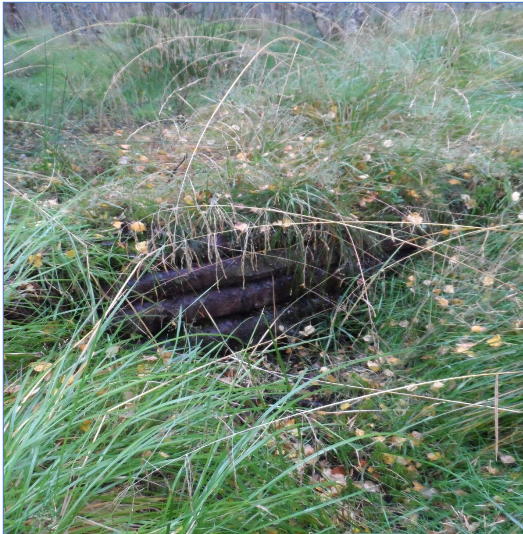
Figure 3: Photo of existing dam structure (local timber with peat infill)
