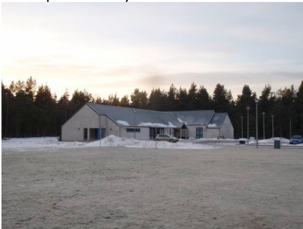
Figure. 4- Boat Community Hall site behind hall
