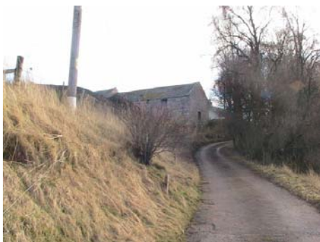
Fig. 2 : Existing watermill structure, with roof of existing residential property in evidence to the rear.
