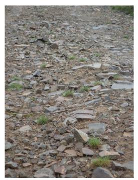
To date the track has been re-surfaced from borrow-pits at Grid Ref NJ315032, NJ314040, NJ 313043 and NJ 313050 with 300 metres of side ditching installed where the track turns at GR 314038. The stone used is of good quality but requires to be compacted using a heavy roller/plate to help seal the surface and form a chamber to shed water. Some fines may be required on the steeper sections though there is evidence of vegetation recovery already taking place (see left).
