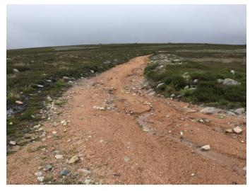
volume of water it has to cope with. Again from here down to the junction with the next track at 57.10534-2.98138 the culvert regime needs to be increased as many of the existing ones have been overwhelmed. This along with the installation of berms should address the problem and protect against future storms.
