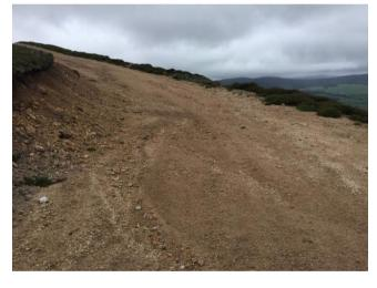
and berms. The existing drainage ditch requires re-vegetating and would benefit from the installation of some stone stoppers to reduce the speed of flow.
