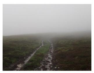
The other section continues North up the ridge. At 57.12685-3.13458 there are 2 gullies that would benefit from the installation of stone fords rather than large culverts. The track continues from here up to the final borrow pit and the end of the previous construction at 57.13222-3.13475. Here the track reverts to 2 deep ruts which are acting as ditches in wet weather. These ruts should be resurfaced and berms installed to slow the flow of water.
