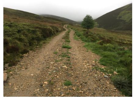
There are sections on the track (see photo) that have a steep exposed bank on the top side of the tracks North spur between 57.12495 – 3.11686 and 57.12528 – 3.11724 (40 m) and also between 57.12577 - 3.11716 and 57.12584 – 3.11602 (70 m) the steep embankment should be reduced in height and vegetated over using borrowed vegetation and turf from the lower slope.
