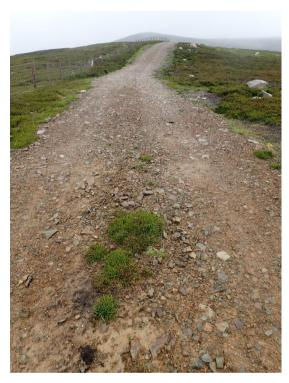
Where sections require extra side-drains to be installed then there will be an opportunity to win material from the ditches. (see Turf lined ditches). The intention would be to "camber" the tracks as much as possible rather than to excavate ditches thus reducing the visual impact of the operations.
