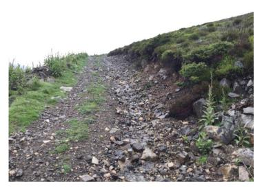
The spoil on the lower side is to be buried and re-vegetated and also used on the upper slope with any large boulders being used in the revetment wall.
