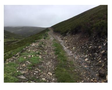
The upper section after the exposed embankment has much more vegetation cover. There is a very small amount of work required on the top side of the track and only requires berms to be installed to reduce the flow of water down the track. There is a turf centre line here starting to establish.
