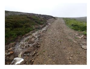
At this point there has been a considerable amount of wash out from the ditch running alongside the track and the installation of culverts every 40m minimum from here passed the 2 borrow-pits at 57.12253-3.13433 and 57.12472-3.13499 up to the fork in the track at 57.12540-3.13505 will prevent this scour happening in the future. Berms should be installed as needed.
