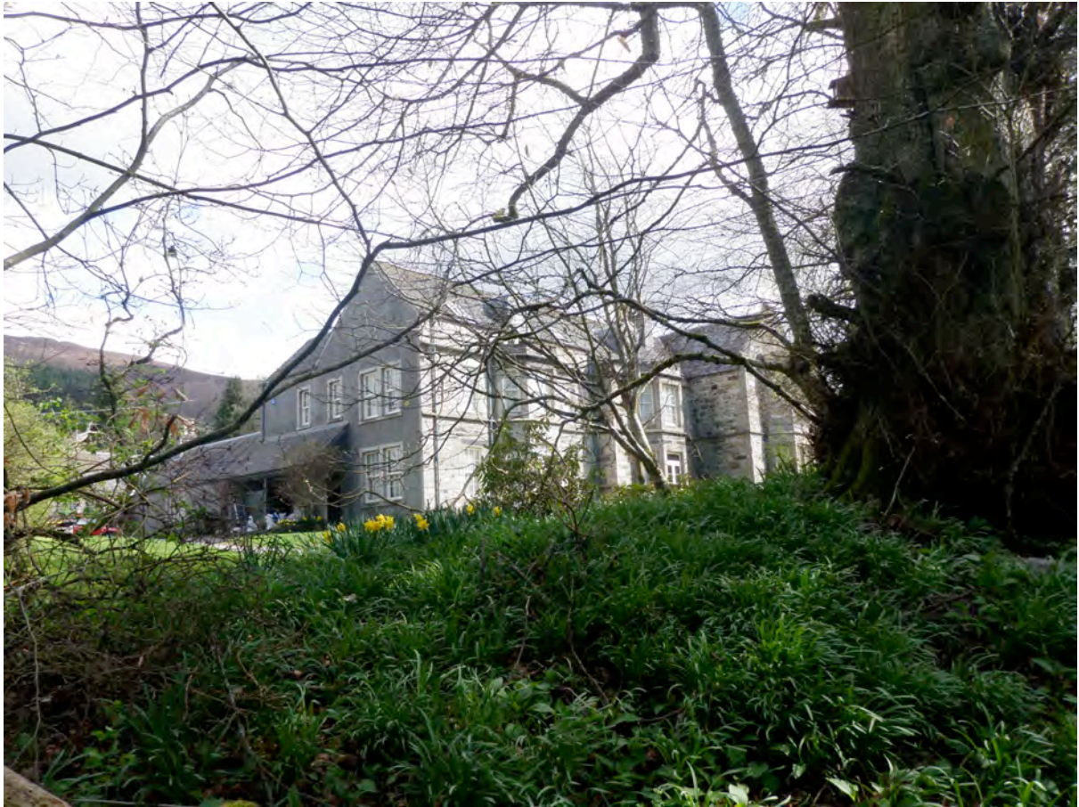
Picture C- View of the house and the staff annex from the locked gate.
