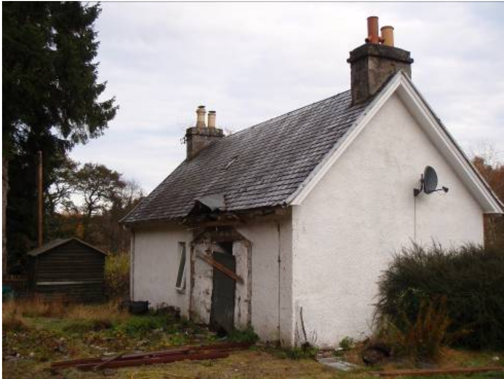
Fig. 3 Rear of Feshie Cottage
