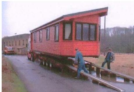
Fig. 4 : method of delivery to site
