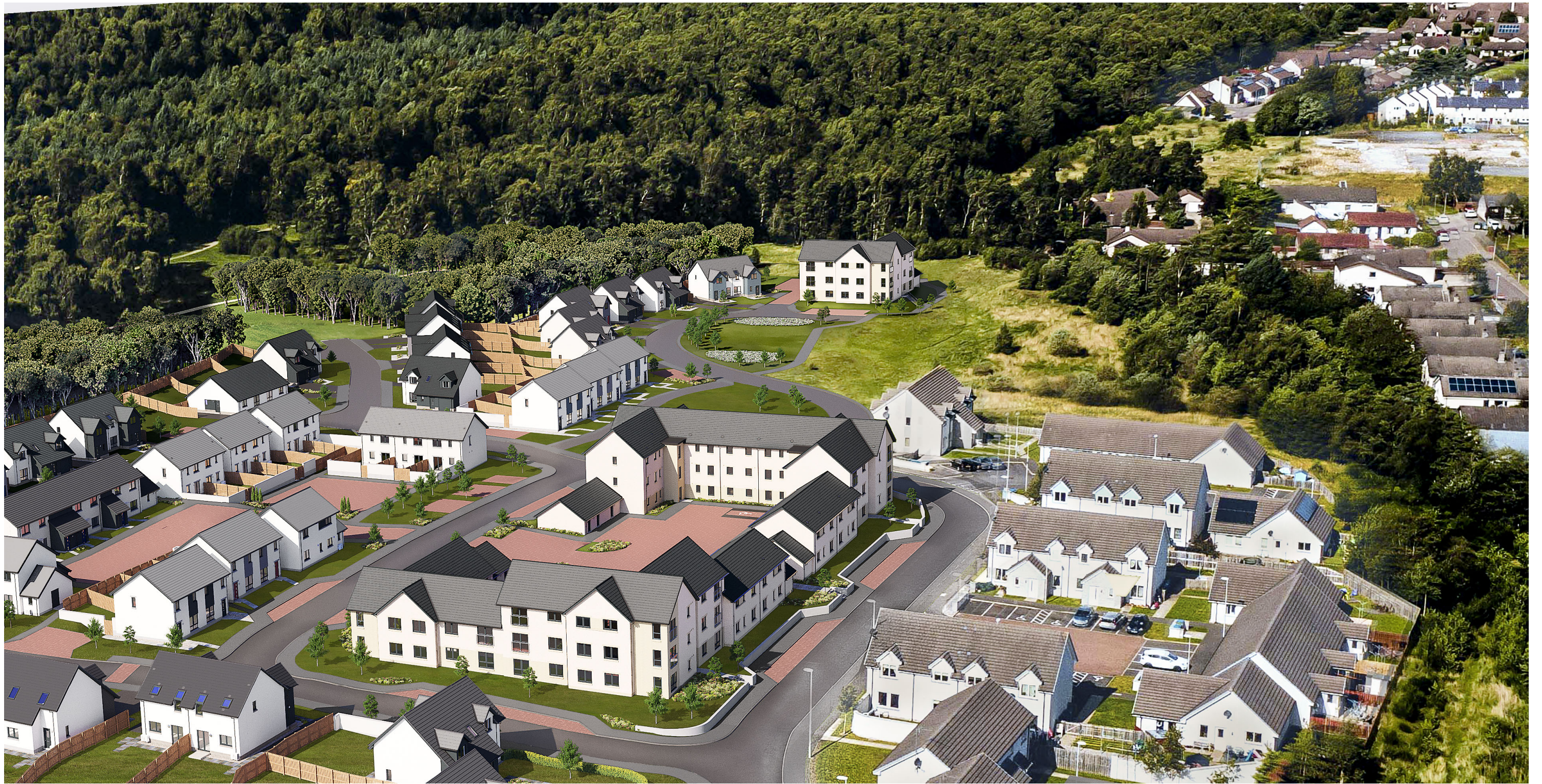
Aerial image looking north with Block 4 in the distance
