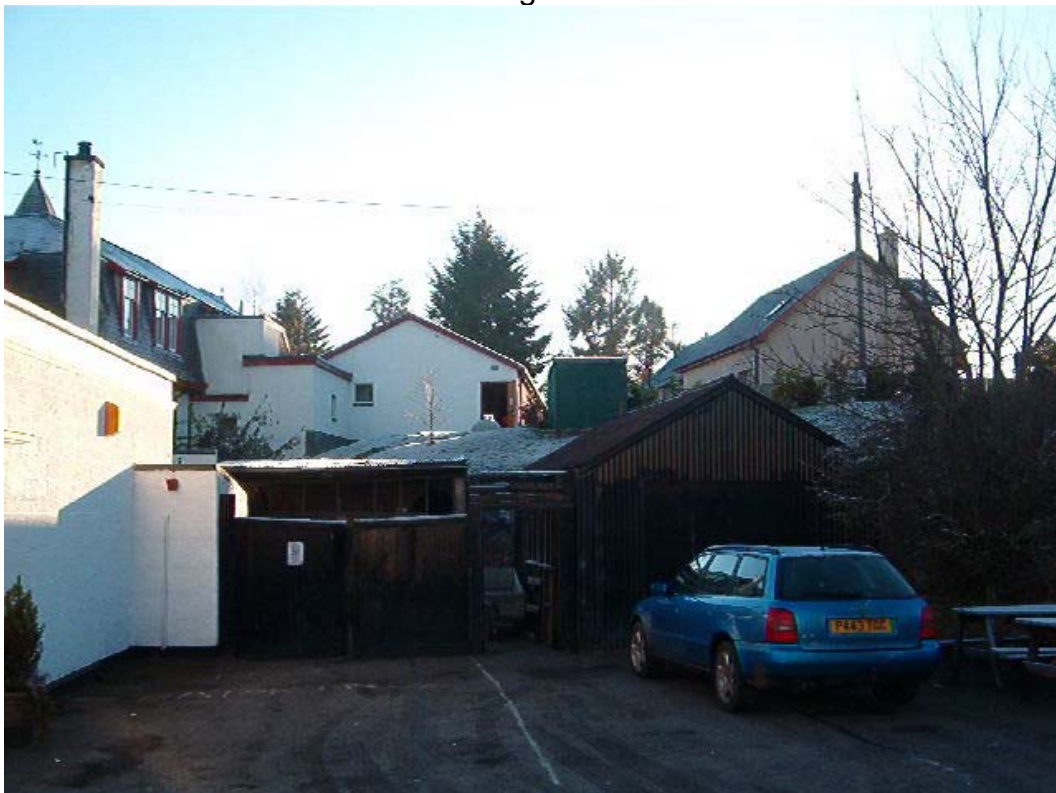
Fig 2 shows relationship between hotel extension to be demolished (centre) and new houses (right) to the west of the site.
