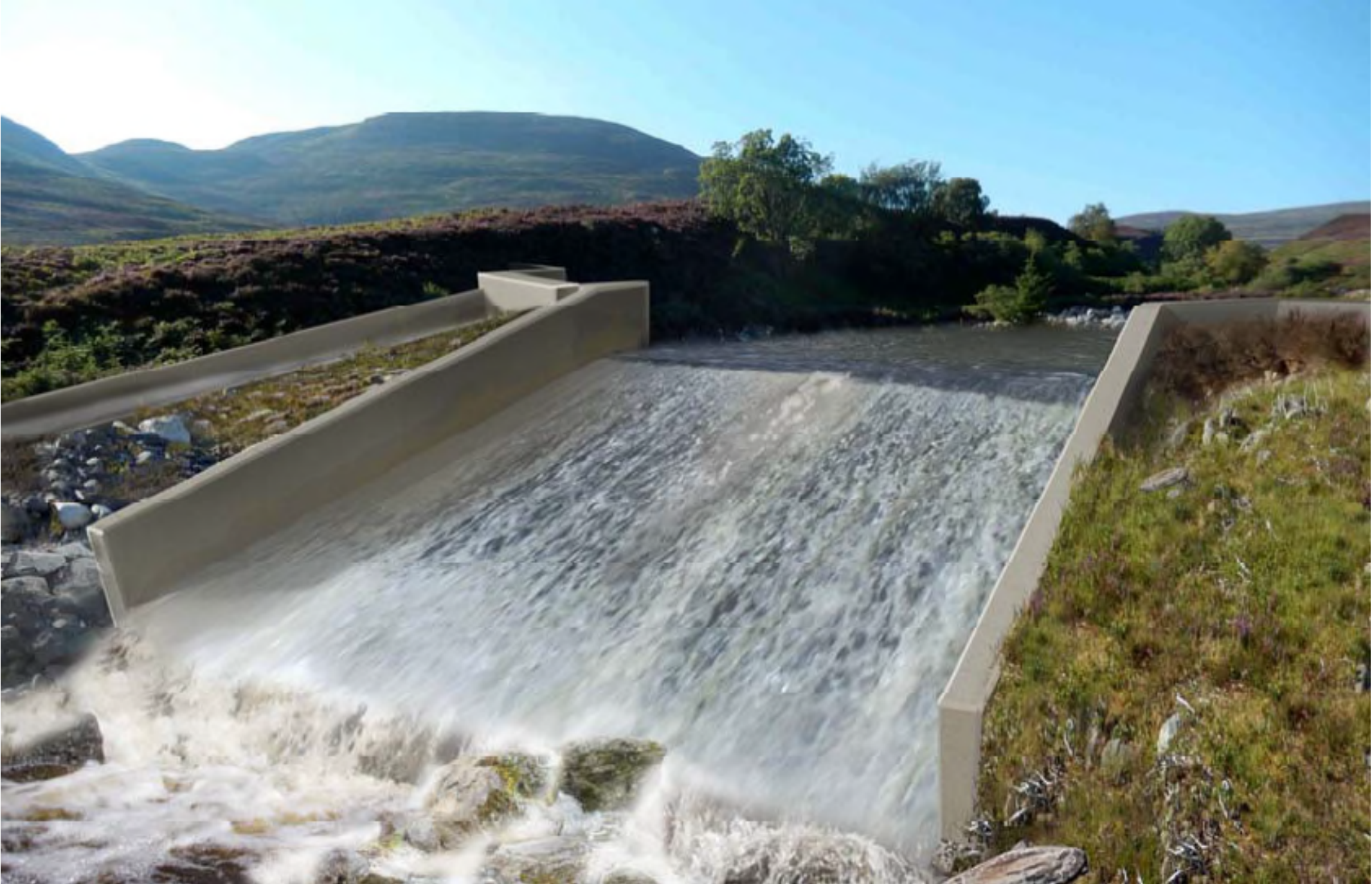
Intake and wing walls at Allt Mhor (visualisation)
