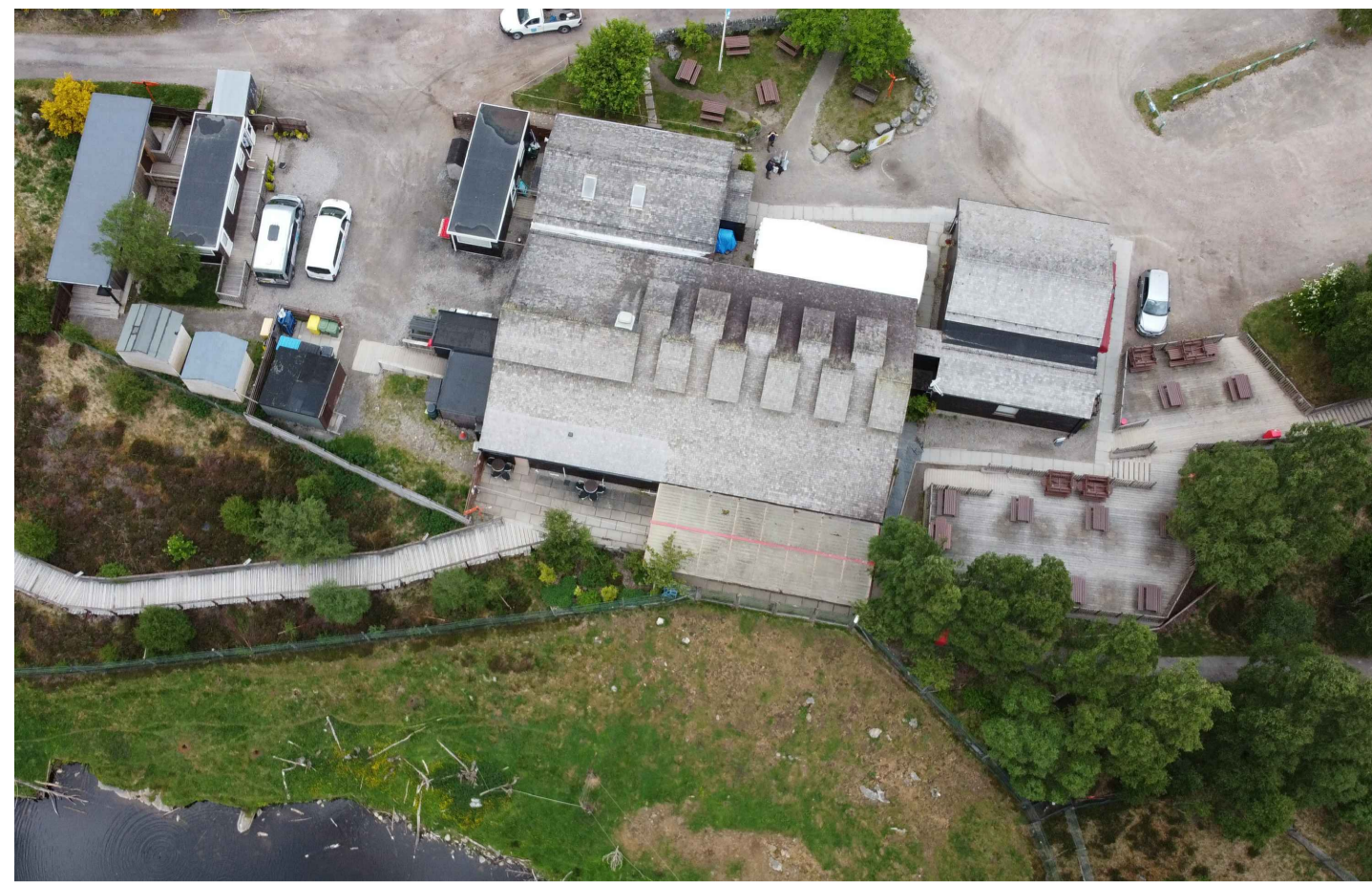
AERIAL PHOTOGRAPH AT THE EXISTING VISITOR CENTRE (nts)
