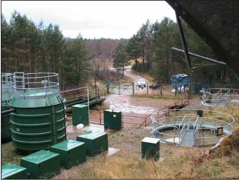
*Fig 3: Photo of the site, taken in a south west direction. The large green structures are the SAF units.*
