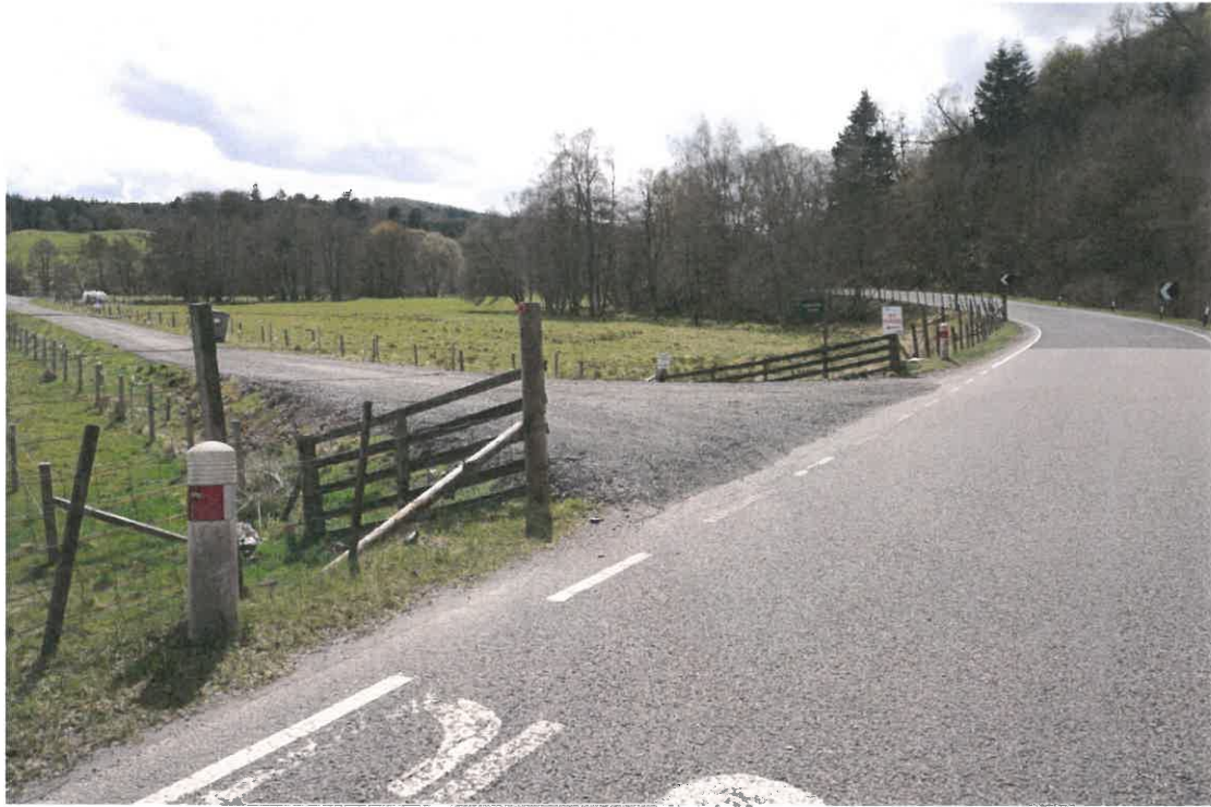
Figure 2: Photo of entrance approaching from the east
