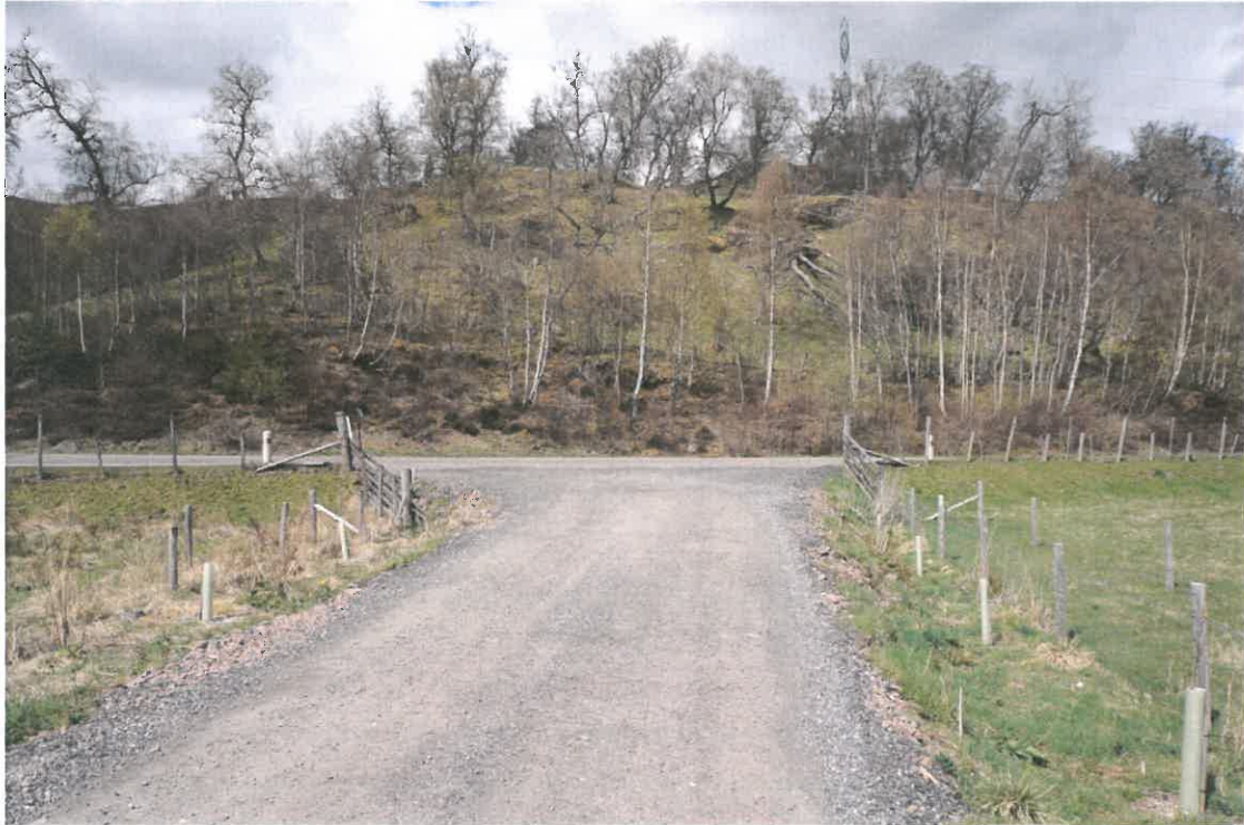
Figure 4: Photo of entrance approaching from the south
