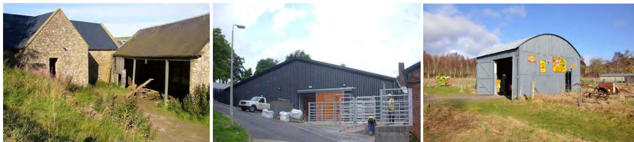
Fig 7. Corrugated/profiled/seamed metal cladding with a generally grey appearance.
