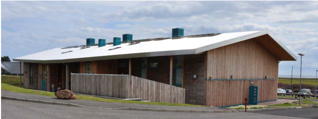
Fig 9. Natural mill finish aluminium roof sheeting and untreated larch cladding greying to a natural colour.
