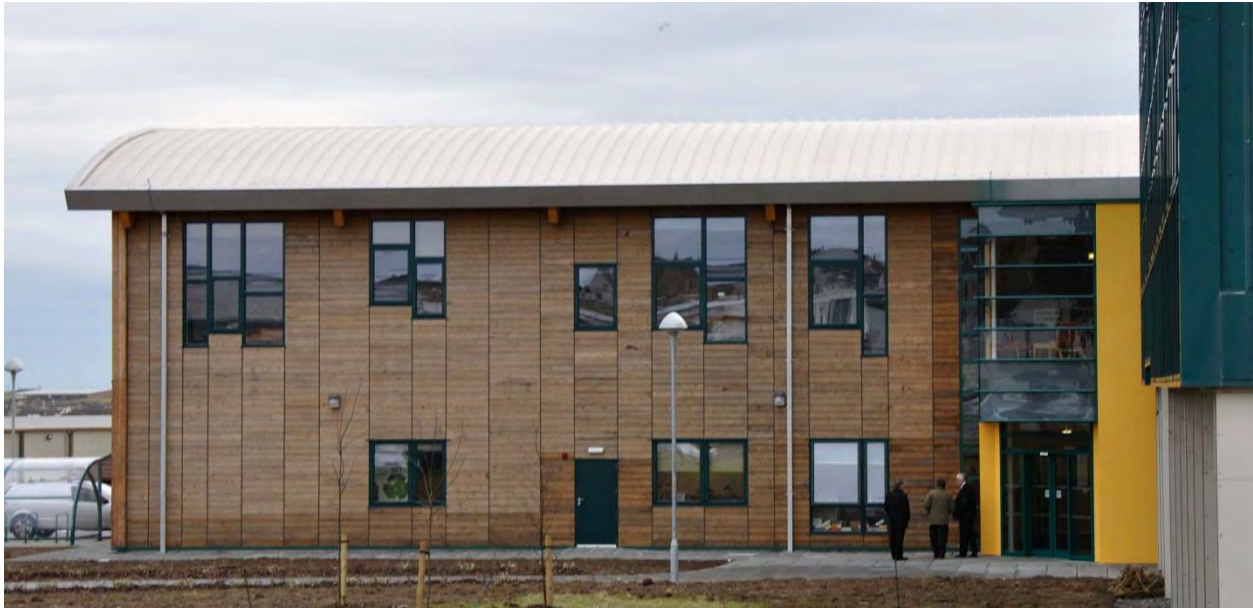
Fig 8. Kalzip standing seam aluminium roofing – greys to a natural finish blending with the sky.
