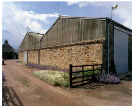
Fig 6. Asbestos roof cladding & timber sidings.
