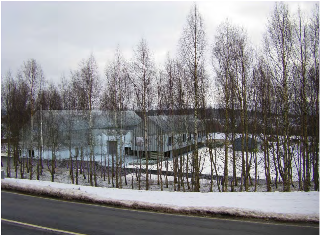
Fig. 1 Photomontage showing proposed building viewed from the A86 at the main entrance to the site.
