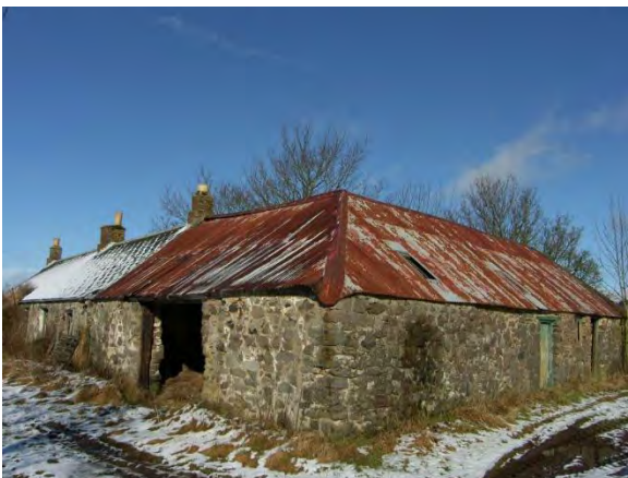
Fig 5. Corrugated tin roof on stone byre.
