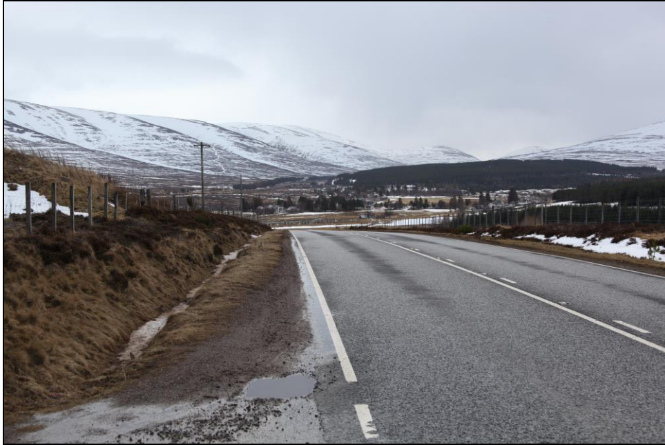
Photograph 1 – View north along the A889(T)
