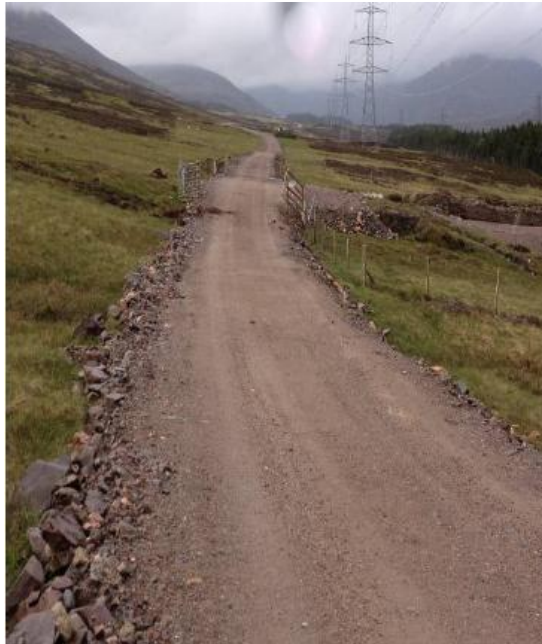
Figure 4: Photos of current floated track (Extract from Reinstatement Report for the Beauly Denny Line Access Track 25 – Ralia Estate)
