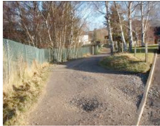
Fig. 3: Existing gravel track
