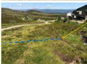
< Image showing view down slope along Allt Chais watercourse bank taken from upper footbridge. End of upper drainage pipeline shown in blue, terminated away from the watercourse with silt trap immediately below HDPE Pipe.
