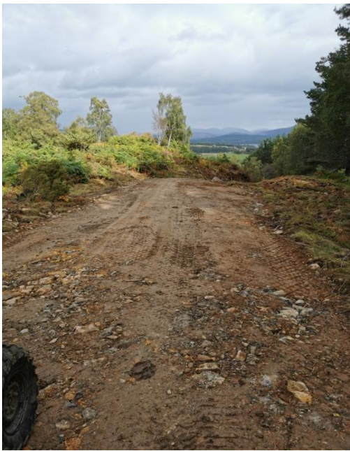
Track Section awaiting final surface
