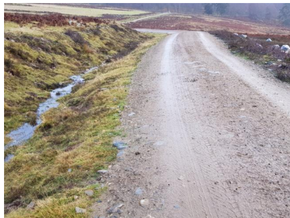
Example of existing hill track construction at Balavil Estate
