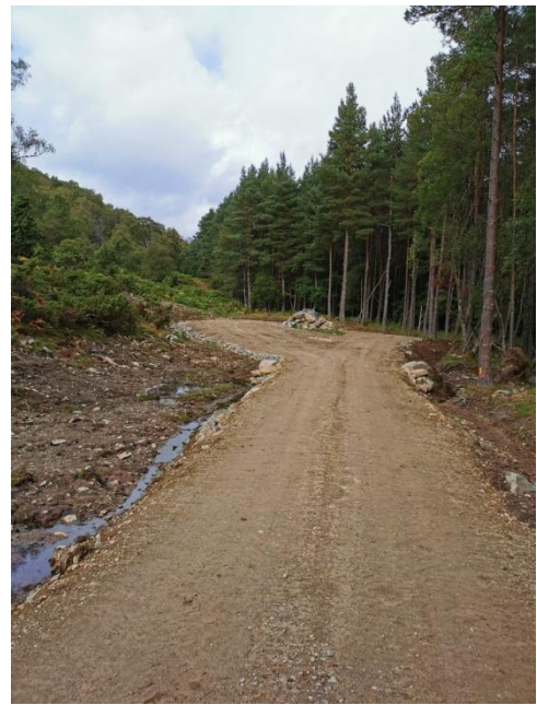
Completed Turning circle (east end of track)
