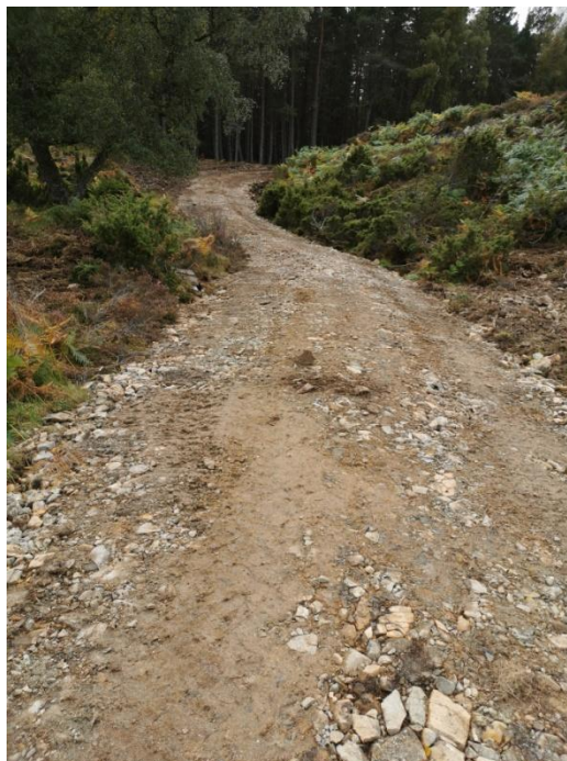
Section of Track awaiting final surface treatment
