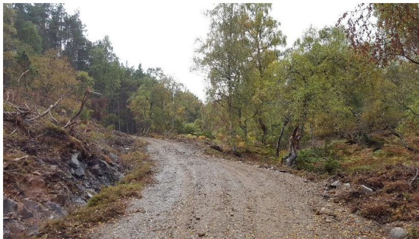
Photograph 9. The constructed track uses the contours of the hill to run between the plantation (on the left) and the semi-natural woodland (on the right).
