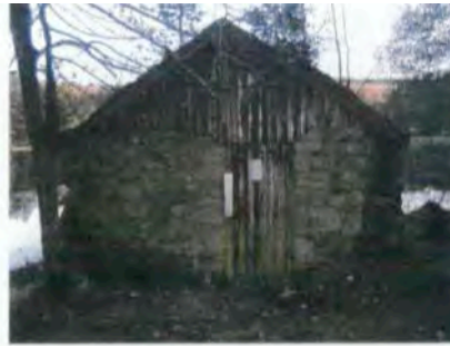
NORTH-WEST GABLE - EXTERIOR
