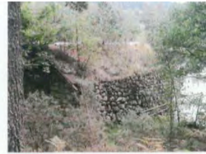
SOUTH-WEST WALL - EXTERIOR
