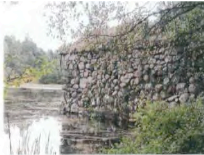
NORTH-EAST WALL - EXTERIOR
