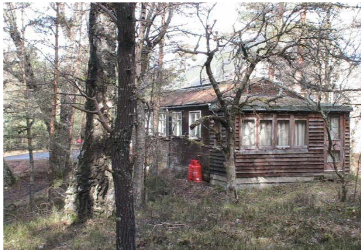
Fig. 4. Existing structure to be replaced
