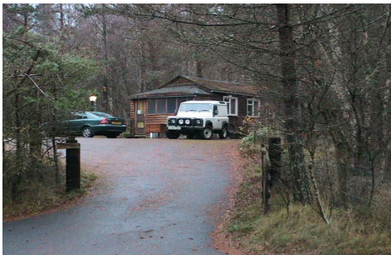
Fig. 3. Existing Structure to be replaced
