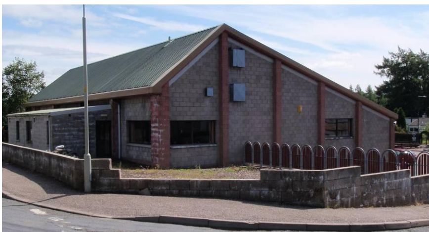
Fig. 2 : example of existing exposed blockwork finish on northern and western elevations
