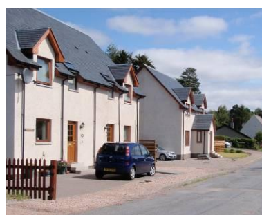
Fig. 5 : Recently constructed properties in Church Terrace
