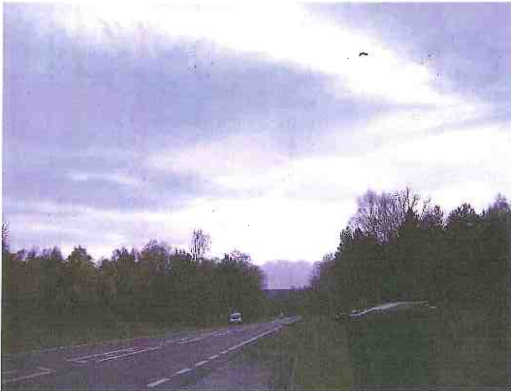
Visibility from existing access looking west at 2.4 metres setback
