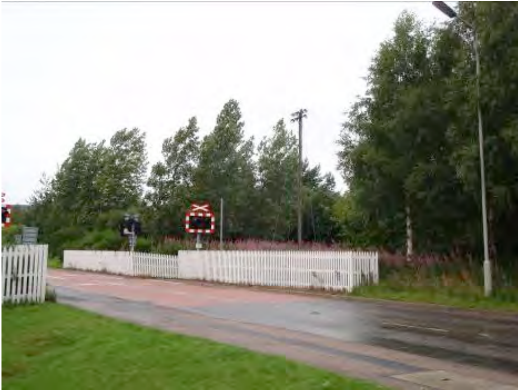
Figure 3 : The site looking North West across the railway line
