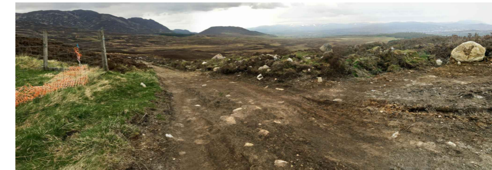
SITE PHOTO: B-B
