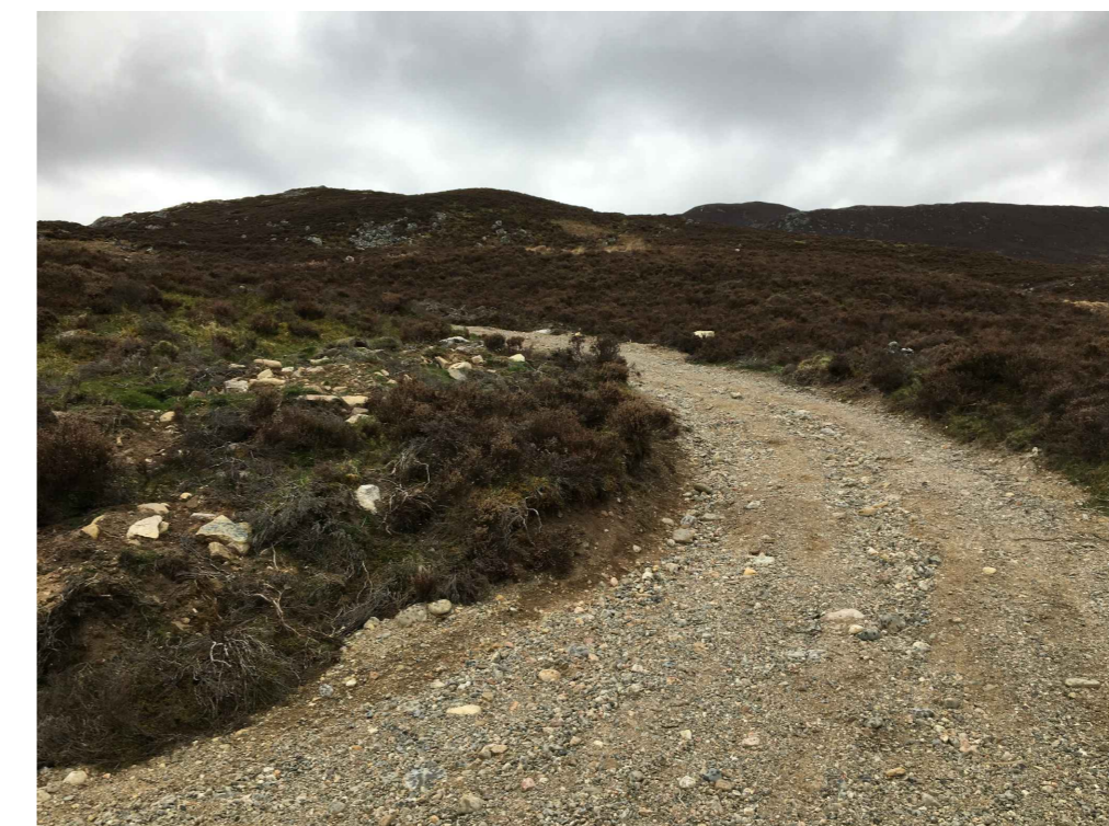
SITE PHOTO: C-C
