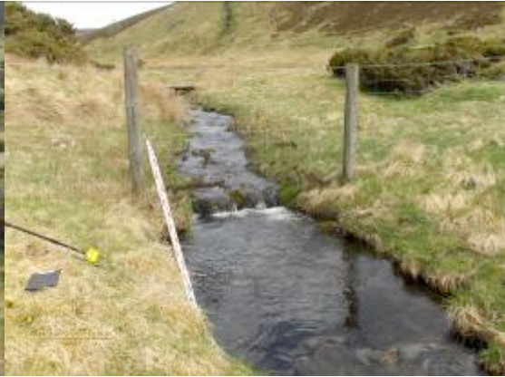
Fig. 3 Burn at site of intake weir
