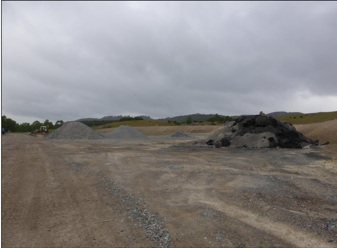
Figure 2 – Site of the proposed temporary plant.
