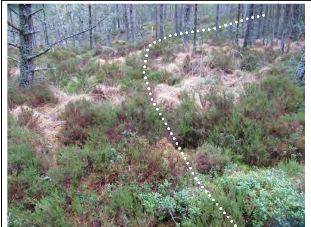
Path is floated on geotextile across 8m of boggy ground and turns right through small diameter pine.
