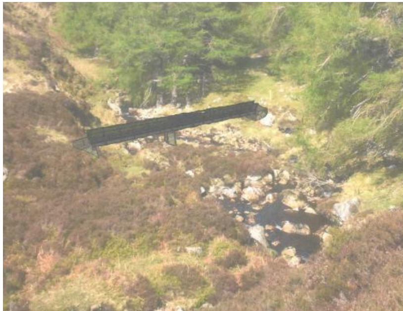
Figure 4: Photomontage of Pipe Bridge (Extract from Drawing No 12018D001-05 11 of 11 Pipe Bridge Photomontage – for information only).
