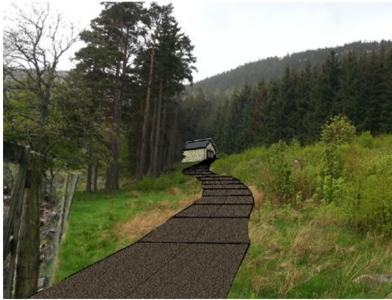
Figure 5: Proposed Turbine House (Extract from Drawing No 12019D001-01 1 of 6 Turbine House Context and Annotations – Laurie - for information only).
