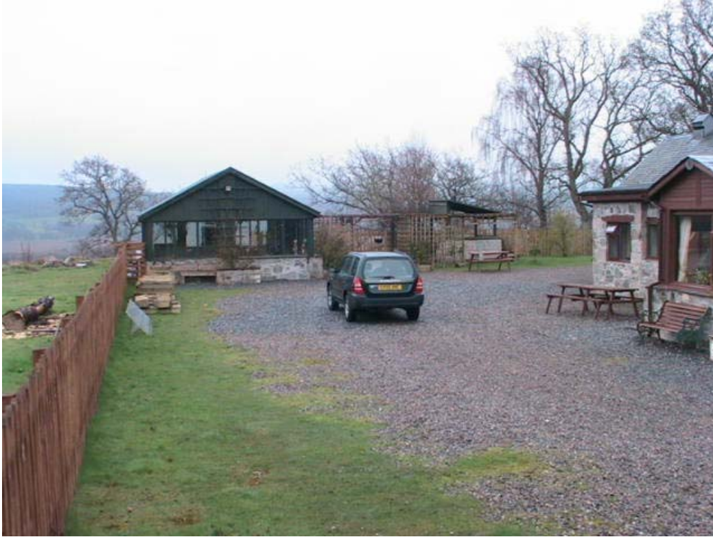
Fig 2 Existing sunroom and pergola area to be converted/extended.
