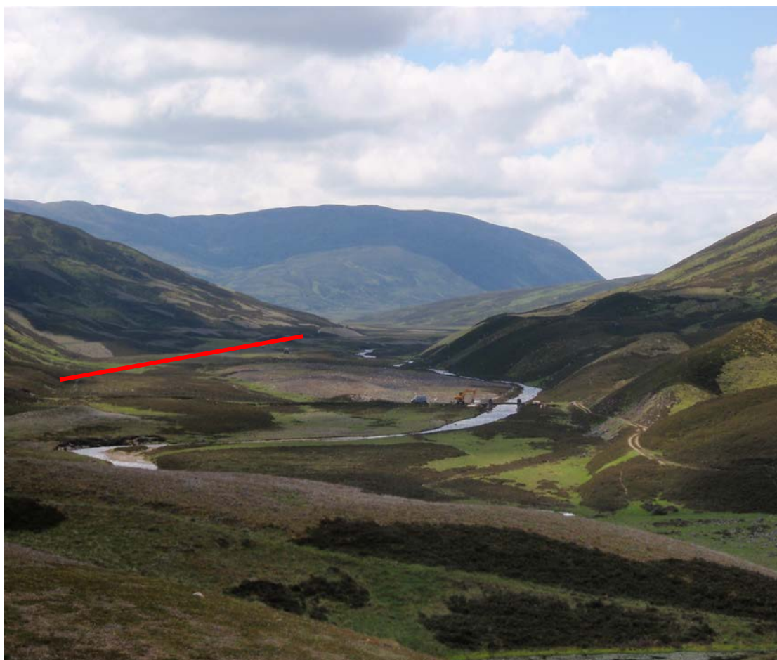
Fig. 2- Site of works area, track alongside left bank of river to be restored, new track (red line) to be on shelf set back from flood plain.
