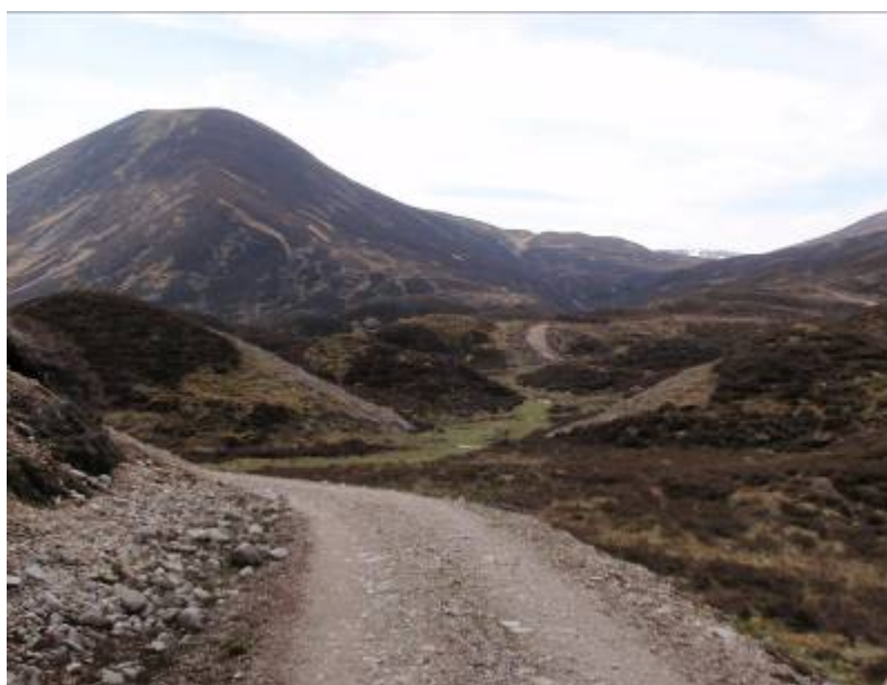
Figure. 2- View of works carried out from track to radio station
