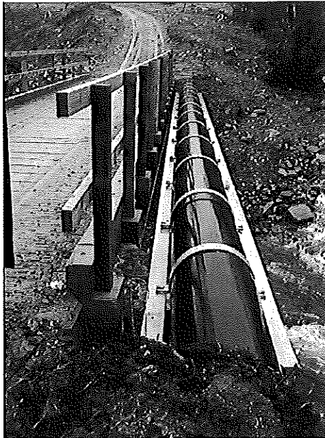
Fig. 6-1 HPPE Pipe Bridge
