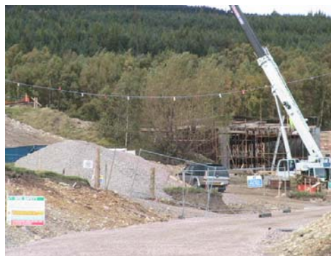
Fig. 2 On-going works at underpass
