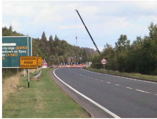
Fig. 3 : southern approach to existing temporary A9 diversion
