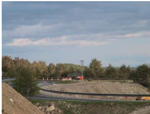
Fig. 4 : temporary diversion of the A9
